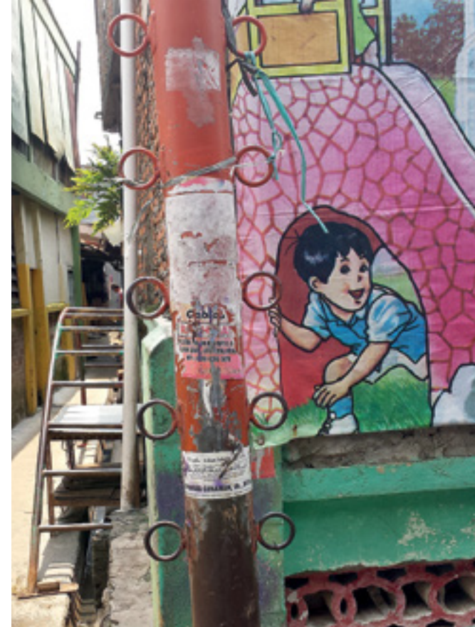
This post is one of several throughout the community of Kampung Melayu. People tie rope lines to the loops, then string rope lines throughout the community that people can grab as they wade through the water during evacuations.
