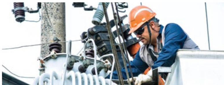
Maintenance in the electric network of AES Eletropaulo
