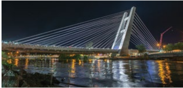
Scenic lighting of the cable-stayed bridge on the South Line 4 Subway – Rio de Janeiro
